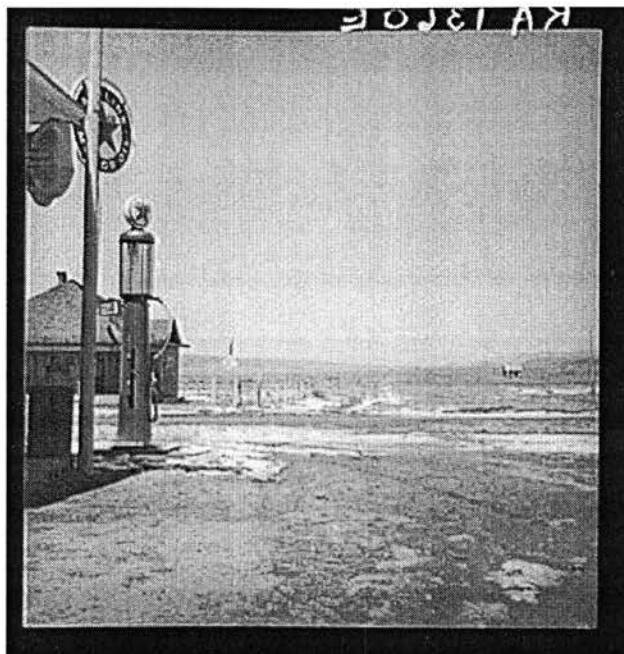
Figure 30- Dorothea Lange, View of the area from the general store. The farm lands purchased lie on the floor of the valley. April, 1936. (LC-USF-34-001360-E)
