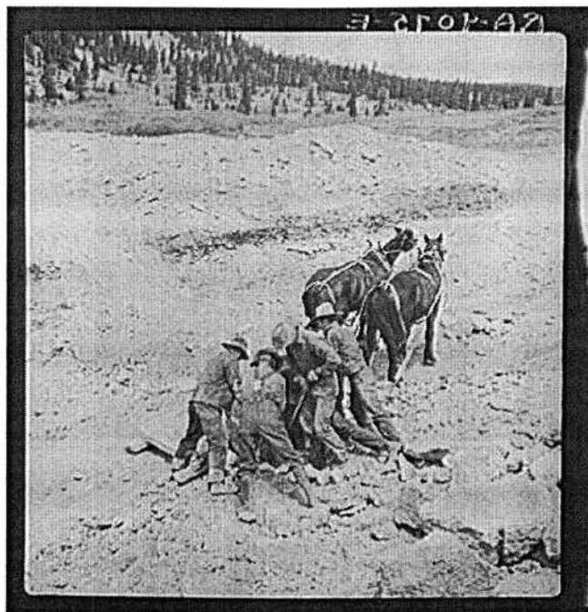
Figure 43- Dorothea Lange, Widtsoe land use adjustment project. Garfield County, Utah. Loading boulder on stone boat, while excavating new spillway of Tropic Dam. May 1936. (LC-USF-34-009075-E)
